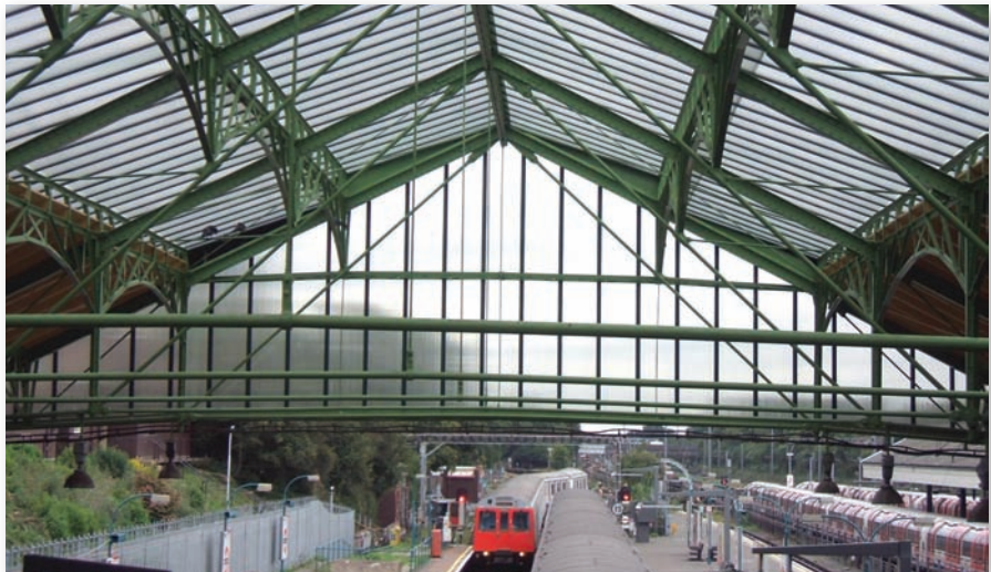
Above: Ealing Broadway station canopy refurbished with Twinfix Multi-Link-Panel NF rooflights
