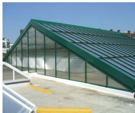
Edgware Station - after with multiwall polycarbonate
