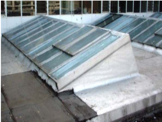
Boots - roof light before
