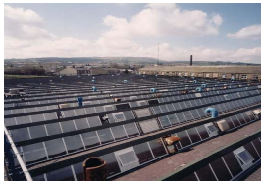
The rooflights at Rolls Royce, Barnoldswick
