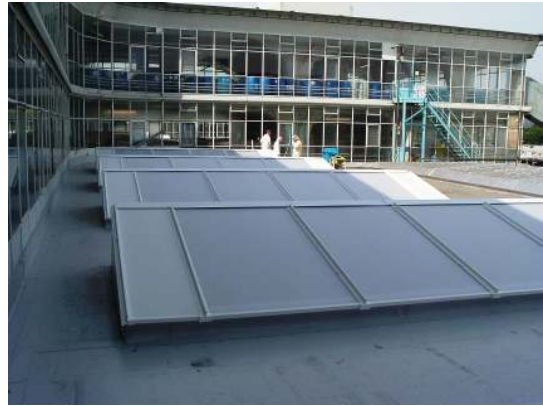
Boots - roof light after
