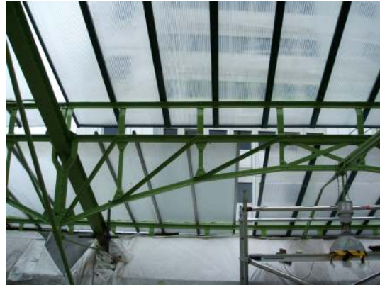
Ealing Broadway – before (bottom left of above photo) & after (bottom right and all of top row)
