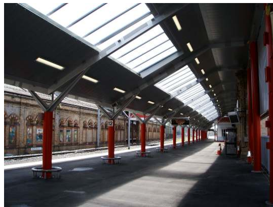
Crewe Station, Platform 12, glazed with Twinfix Multi-Link Non-Fragile pre-assembled polycarbonate panels
