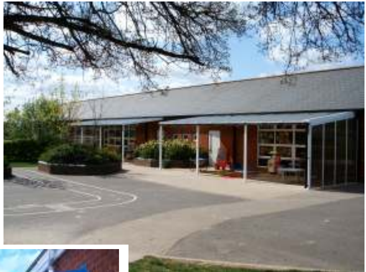
White framed lean-to with vertical in-fill panel glazing to one end to help provide shelter from the prevailing wind
