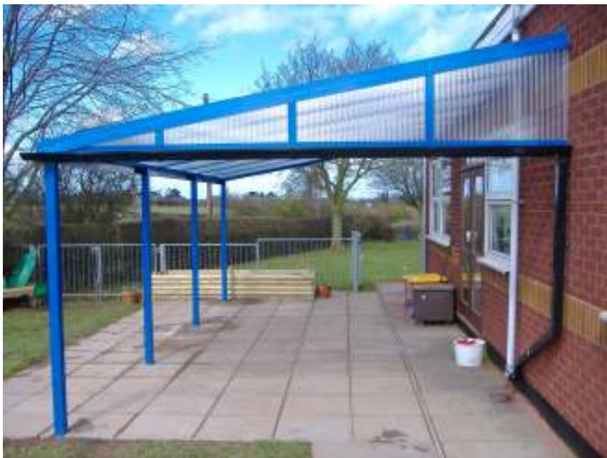
Blue framed canopy with infills across the top to help cut down on rain entry
