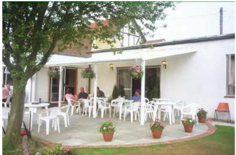
Lean-to smoking shelter glazed with clear multiwall polycarbonate fitted into a white powder coated frame
