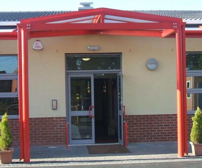
Powder coated aluminium frames, glazed with polycarbonate non-fragile roof panels
