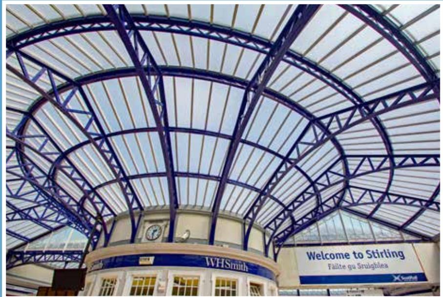
glazing the 2,440 square metre roof, inspection, repairs and painting of the supporting structure as well as relining cast iron gutters and cleaning downpipes, all at a total cost of £2.5 million. The design and execution of this work was part of the station framework contract which Network Rail Scotland had awarded to Story in 2014.
