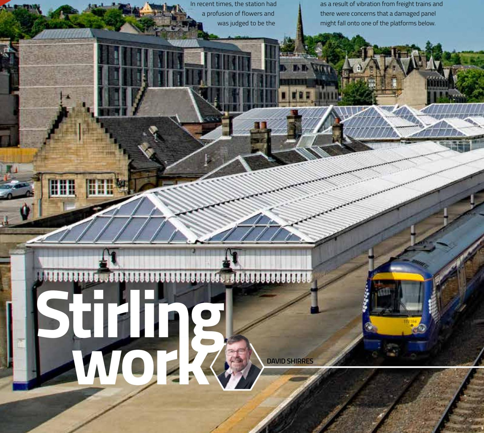
Although the Makrolon sheets used were a Georgian-wired cast-effect polycarbonate which is virtually unbreakable, Stirling City Council's planners were not convinced. Hence it took two years for Network Rail to obtain planning permission to re-glaze the Category A-listed Stirling station.
