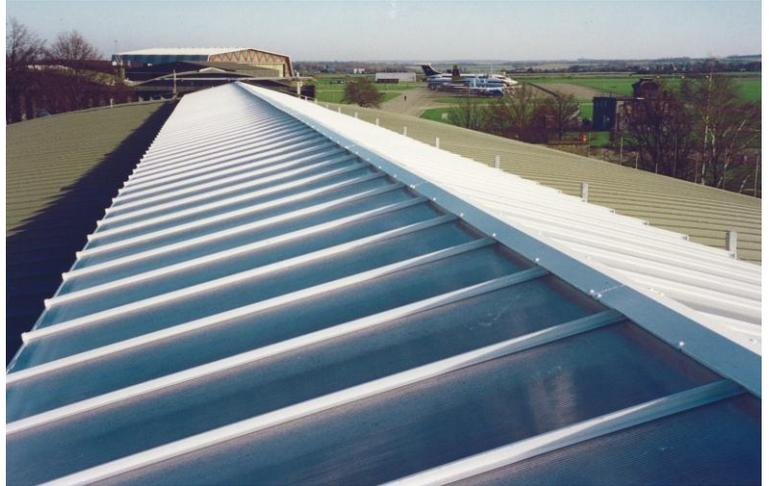
Polycarbonate is available in a variety of thicknesses and tints to allow for effective control of light and heat transmission. Multi-Link-Panels are fitted as northlights over classrooms, workshops, warehouses and railway depots in new-build projects or to replace failed corrugated GRP and Georgian wired glass. Multi-Link-Panels are manufactured to size for each individual project.
