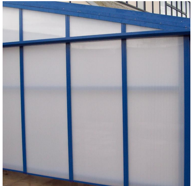
16mm Multiwall Fluted Opal polycarbonate glazing
