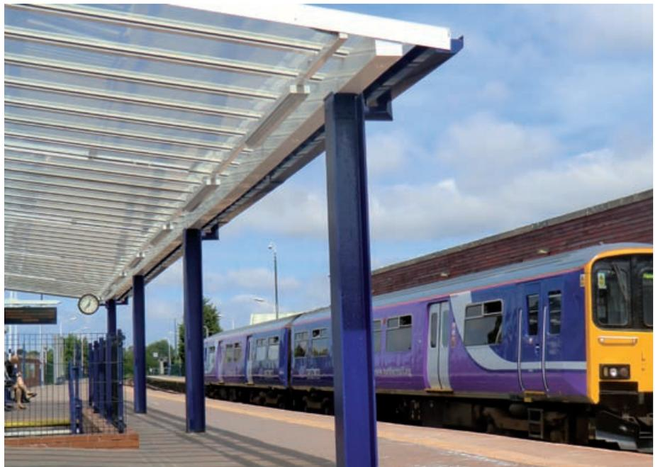
The Twinfix Multi-Link-Panel NF fitted with the following glazing has been tested to the HSE's recommended test (ACR[M]001:2011) and they all pass with a 'B' designation.
