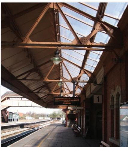
**Stratford station recently refurbished with Multi-Link-Panels NF fitted with aluminium sandwich panels on the left and 25mm multiwall polycarbonate glazing on the right**
