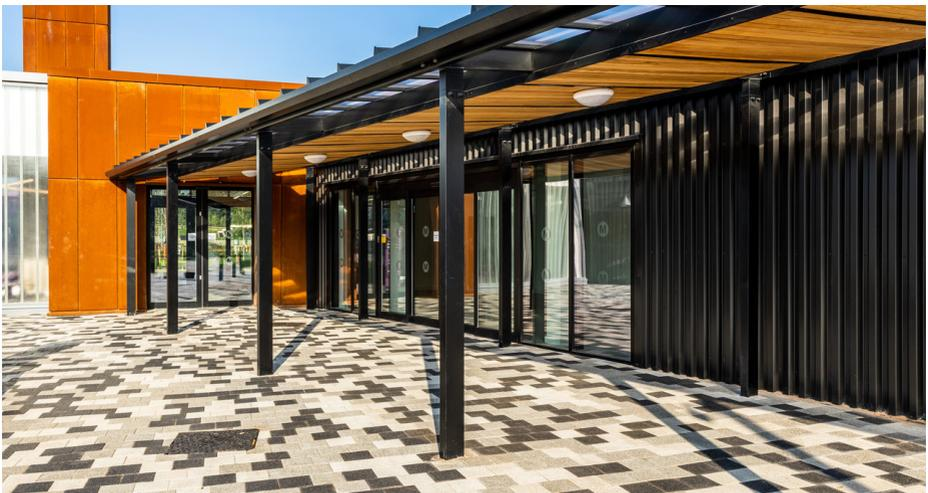
All of these roof structures are made from our Multi-Link-Panel Non-Fragile roof panel system that conforms to the HSE's recommended drop test for roofing assemblies ACR[M]001:2019, and passes with a 'B' designation. Class B is the best result that polycarbonate can achieve.
